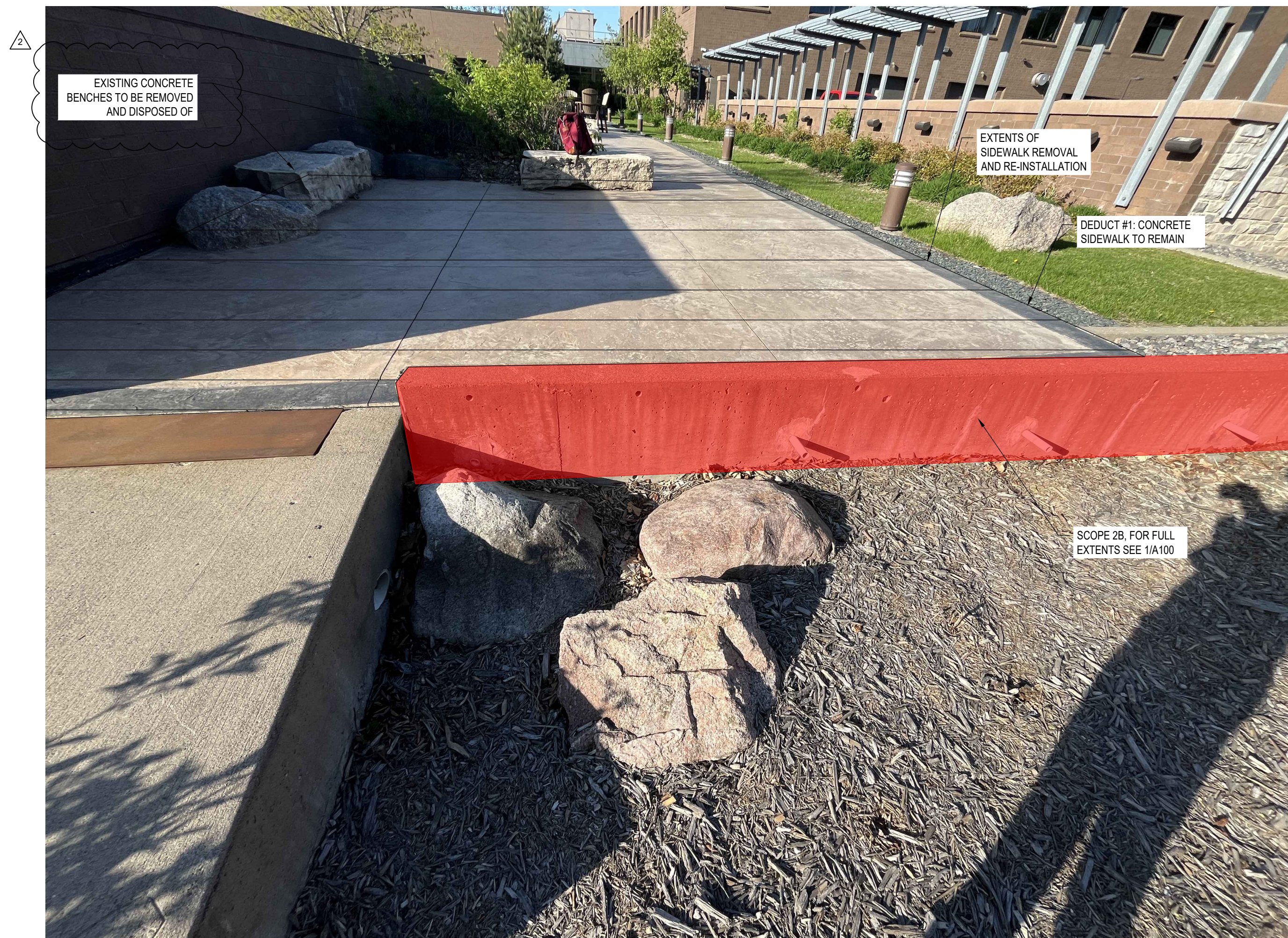
2 SCOPE 2A AND CONCRETE SLAB REMOVAL EXTENTS A500
