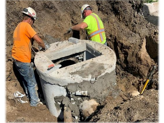
Storm Sewer Installation & Stormwater Management
