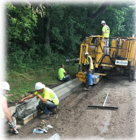
Concrete Curb & Gutter Installation
