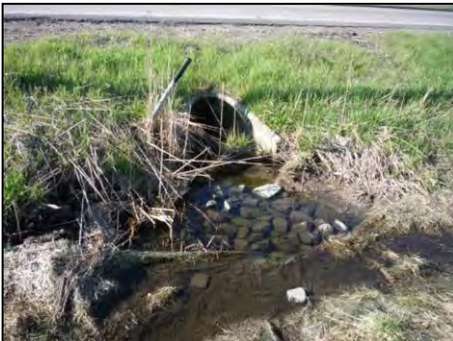
**Figure 3.3. 24 inch Reinforced Concrete Pipe.**
