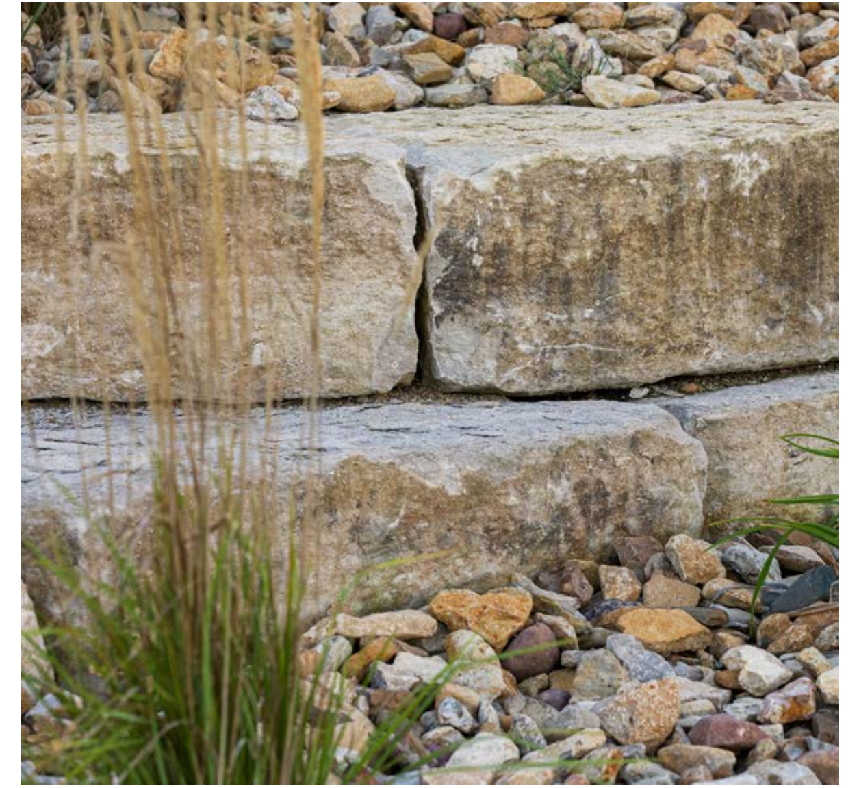
LIMESTONE RETAINING WALL
