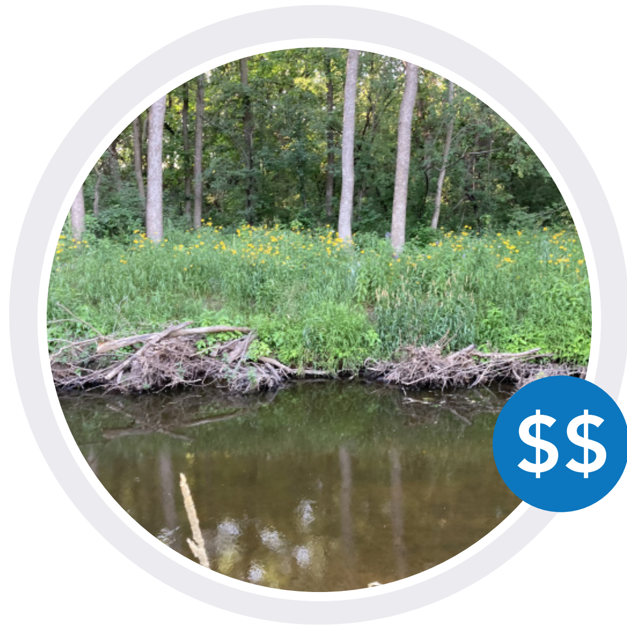
Bank stabilization with bioengineering methods
