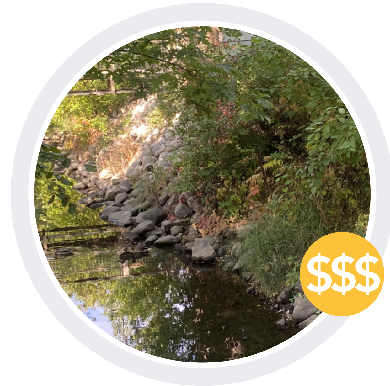
Bank grading with riprap and vegetation establishment
