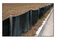
fencing on the downhill side of the filter fabric. Bury bottom 2" of wire fencing. Stake with metal posts, driven a minimum of 12" into the soil. Make sure metal posts are no more than 4' on center.
